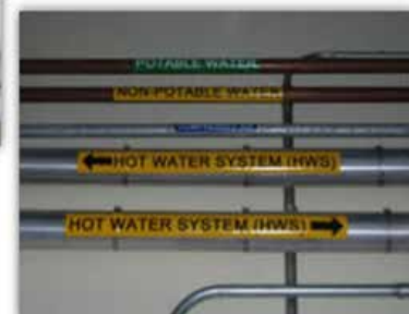
Colour coding of water pipes to avoid contamination
